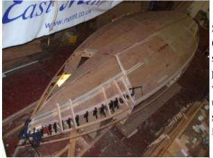
She was built during the early part of 2009 for the Customs House "Coat for a boat Project". Picture shows the hull about half way through being panelled. The were 40 panels in the completed boat which was made in 4 sections so that she could go upstairs in the exhibition room. Once installed there she was covered in knitting and did look impressive.
